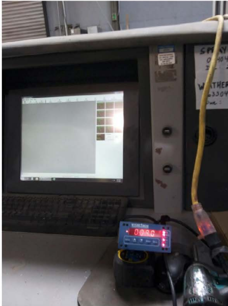
Photo No. 5 Instrumentation
